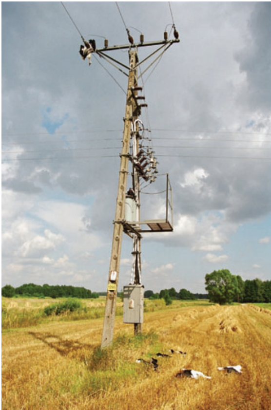
Figure 1 An electricity pole before (left) and after (right) technical modifications (indicated by an arrow) to reduce electrocution of birds. Note the five electrocuted white storks on the ground, and a further one on top of the pole, in the first photograph.
